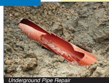
Underground Pipe Repair
