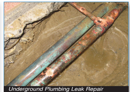
Underground Plumbing Leak Repair
